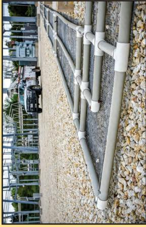
If a snake manages to get past the barriers outside a substation, it still has to contend with electrified wires between PVC pipes that surround equipment. (Sarah Beal photo)
