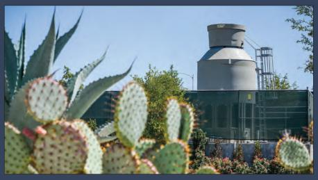
A large gray water-cooling tower connects to the geothermal system that heats and cools multiple homes in Whisper Valley. The cool water in the tower is used on extremely hot days. Water flows through the grid of pipes deep underground that are connected to a geothermal heat pump in each home's attic. The constant temperature below ground provides cool air in summer and warm air in winter.
