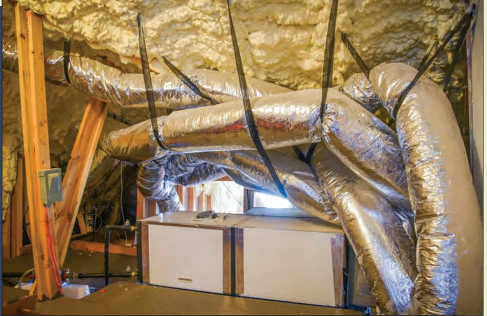
Attics in Whisper Valley are insulated with spray polyurethane foam, which seals the space and reduces unwanted humidity, mold, pollen and air infiltration. The box in the center houses the home's geothermal pump, which transfers the warmth or coolness of the water into air that will warm or cool living spaces.
