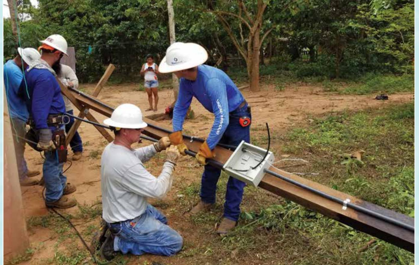
CoServ Electric's Christopher Hammonds, kneeling, and Bluebonnet's Kasper, right, build a meter loop, the conductive wires that connect a meter to a home.
