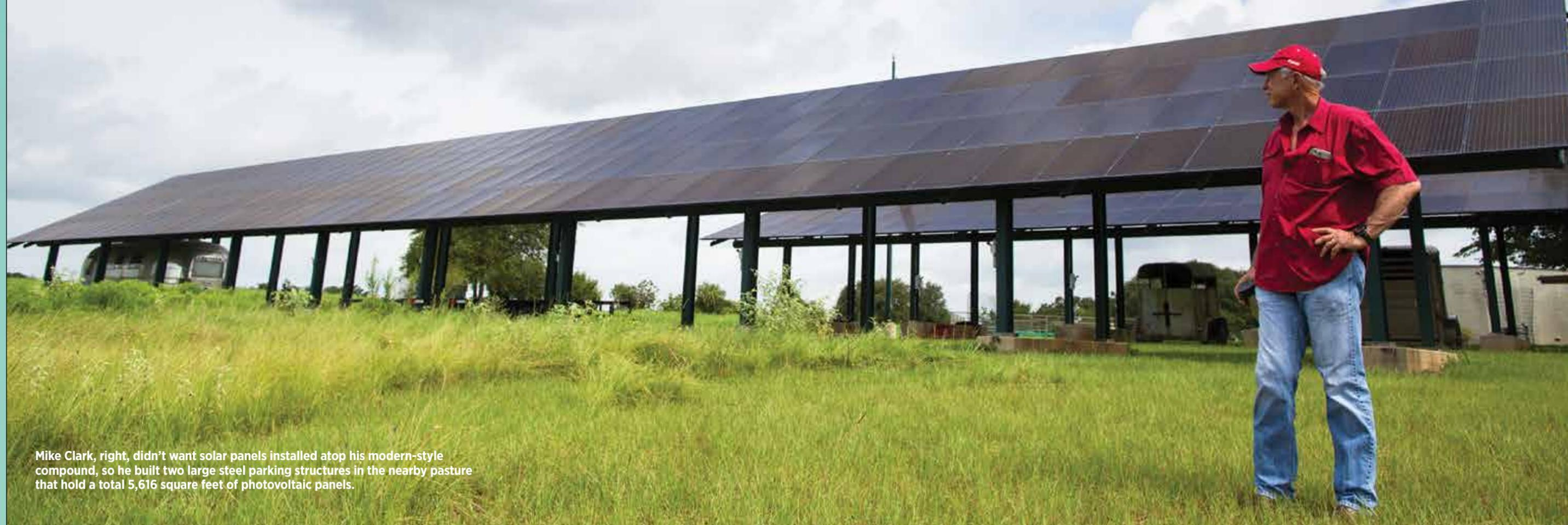
Mike Clark, right, didn't want solar panels installed atop his modern-style compound, so he built two large steel parking structures in the nearby pasture that hold a total 5,616 square feet of photovoltaic panels.
