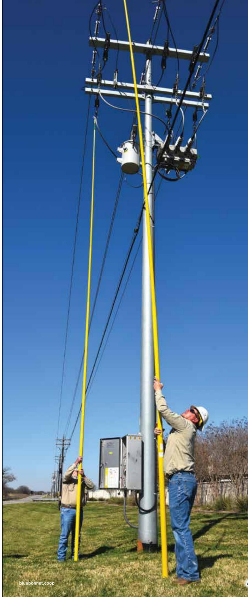
**LEFT:** Gholson, left, and Moerbe use the same hot sticks to close the circuit after a successful test of the new system. **BELOW:** Bluebonnet field operations employee Chad Siegmund monitors the distribution automation equipment to ensure the equipment is functioning properly.
